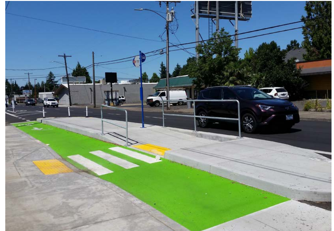
NE Halsey St and NE 111th Ave
