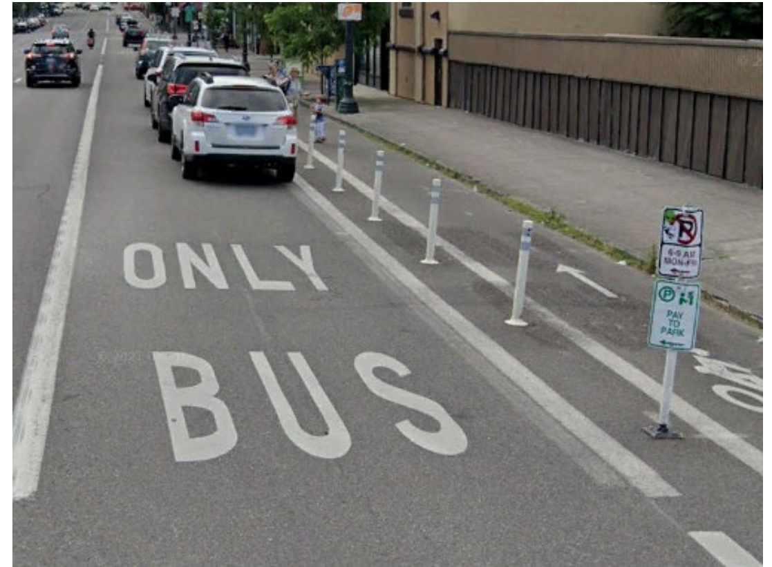
Parking lane along SE Morrison St converts into bus-only lane during morning peak hours.
